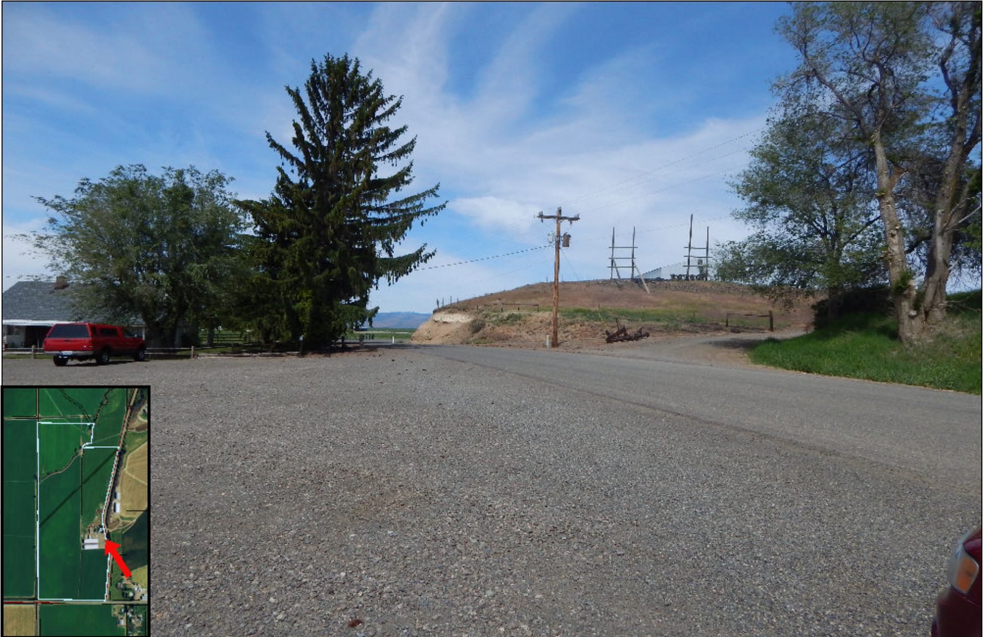
CU-15-00006 Iron Horse Solar Farm
