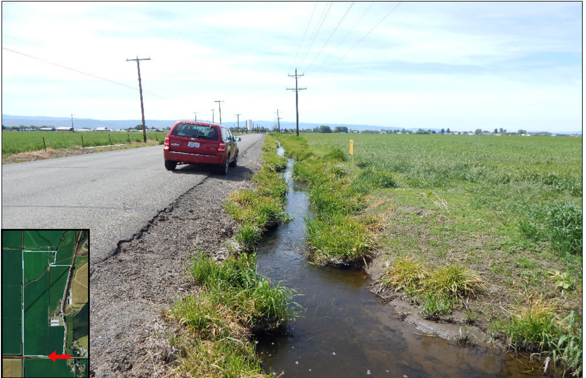
CU-15-00006 Iron Horse Solar Farm
