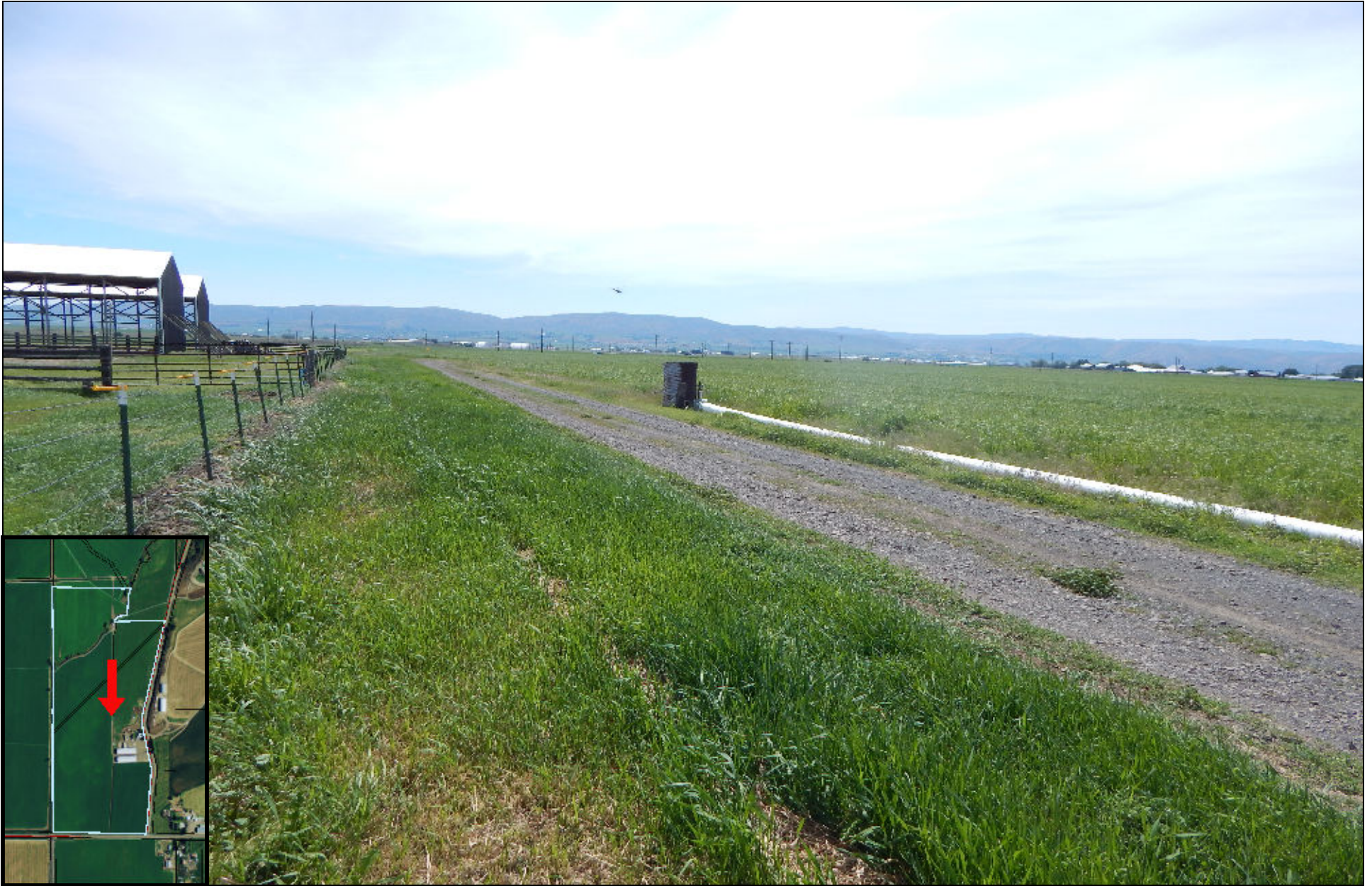
CU-15-00006 Iron Horse Solar Farm
