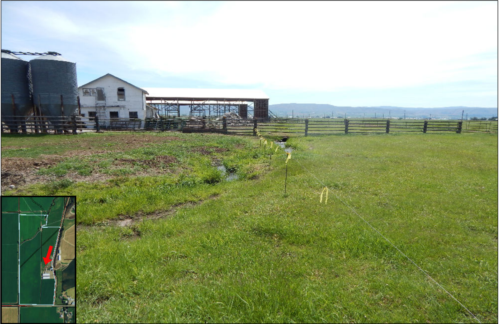
CU-15-00006 Iron Horse Solar Farm
